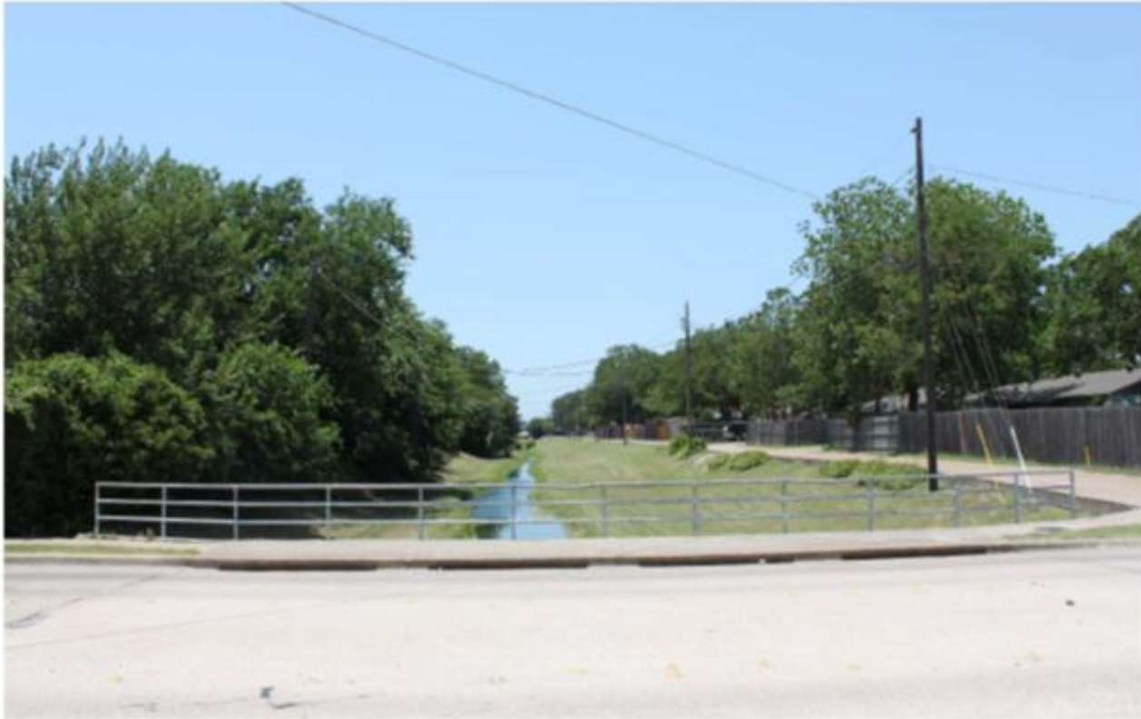
Existing Condition – Westward View
