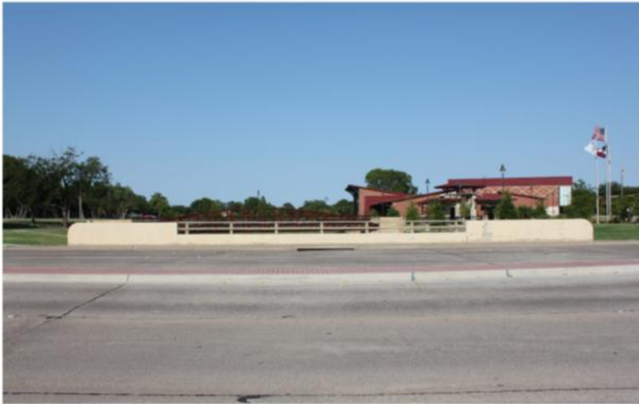
Existing Condition – Eastward View
