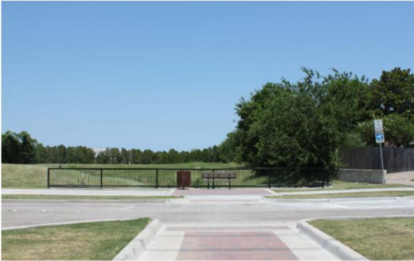
Existing Condition – Eastward View
