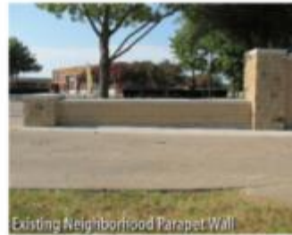
Existing Neighborhood Parapet Wall
