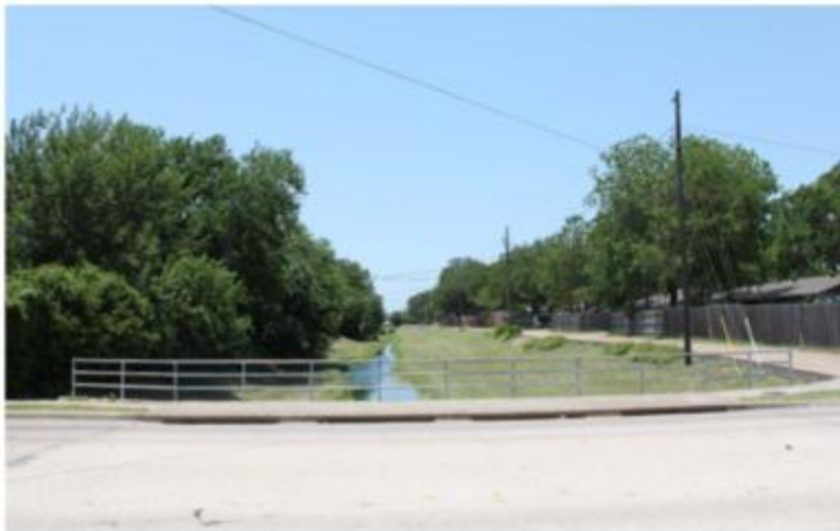
Existing Condition – Westward View
