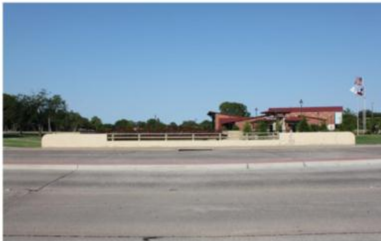
Existing Condition – Eastward View
