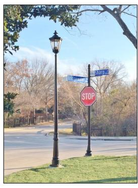
Decorative Traffic Poles must be 4 inches in diameter, constructed with .125 inch wall thickness aluminum tubing and finished in a durable polyester powder coating.
