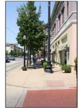
Lighting and ADA Ramps
