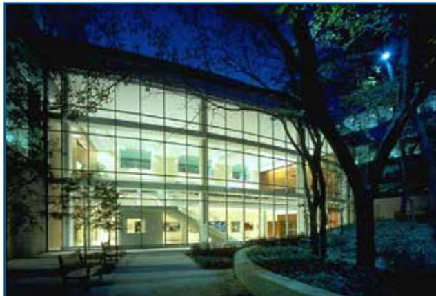
Corporate Office Building
