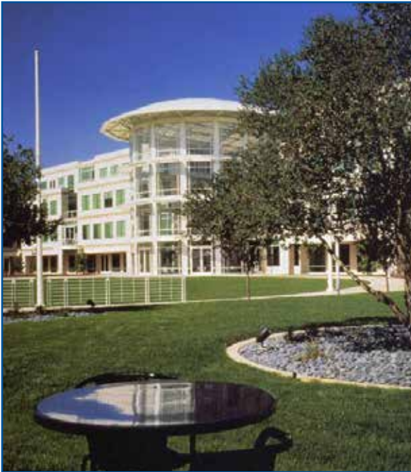
Corporate Office Building
