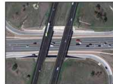
Protected pedestrian access under Central Expressway
