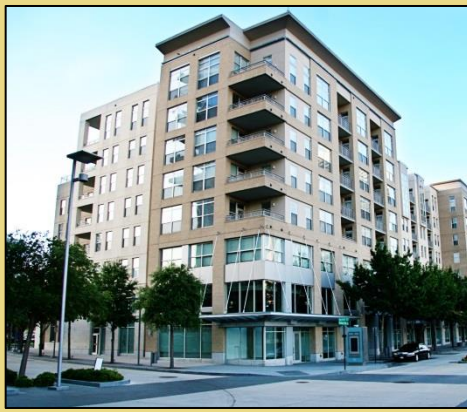
Mixed residential building east of U.S. 75
