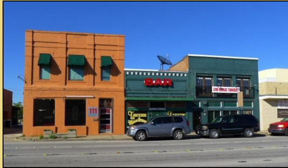
Existing buildings on north side of Belt Line Rd./Main St.
