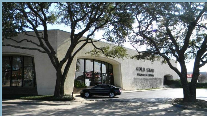
Existing appliance and lighting business – SE corner U.S. 75 and Rayflex Dr.
