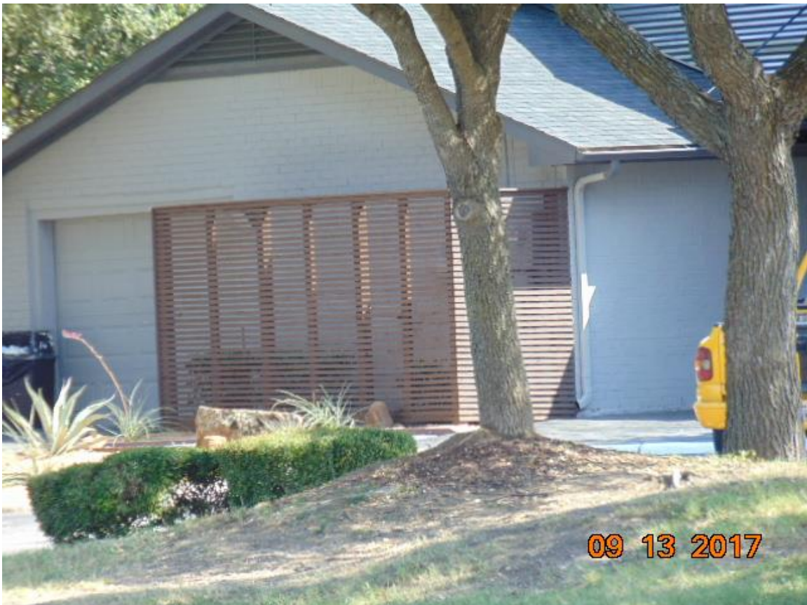
CLOSE UP VIEW OF SCREENING FENCE
