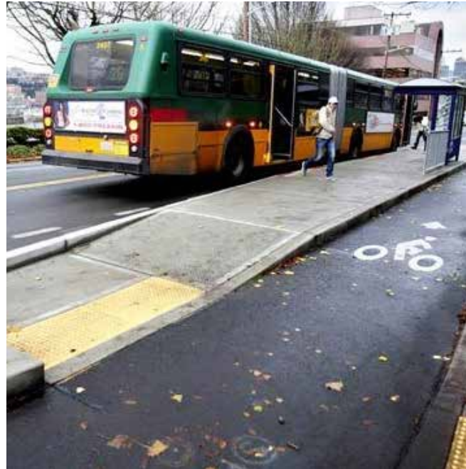
Example of floating bus bulb and bike lane
