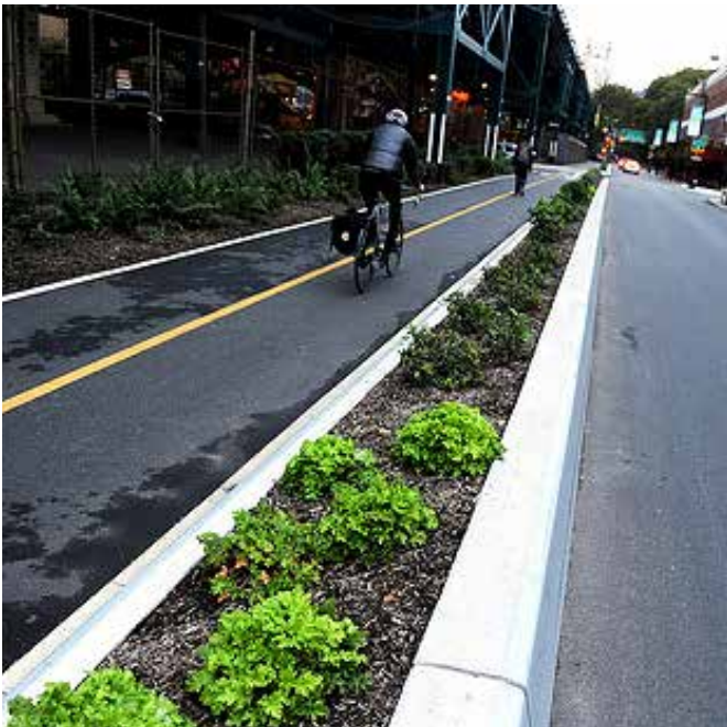
Example of two-way cycletrack
