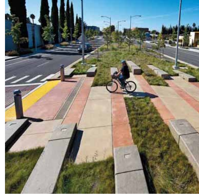
Example of enhanced crossing with median refuge
