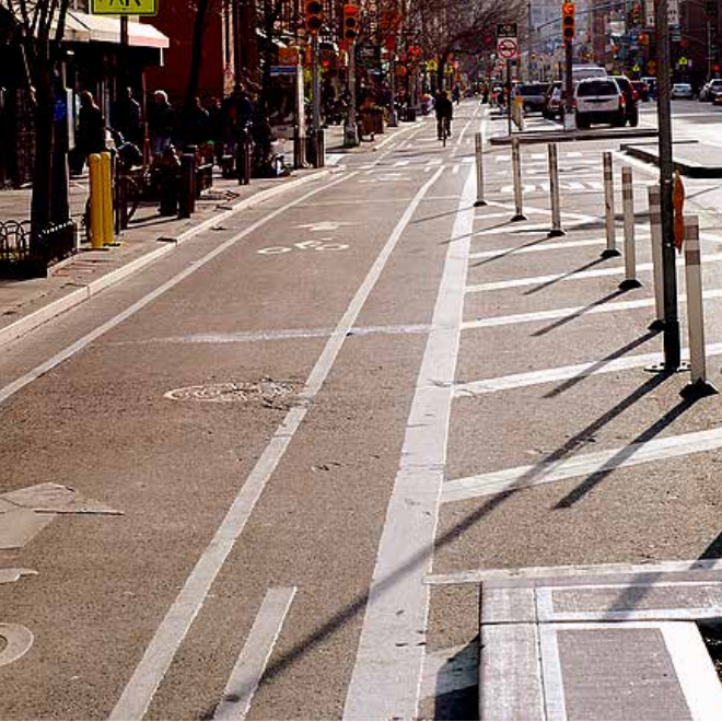
Example of buffered bike lane
