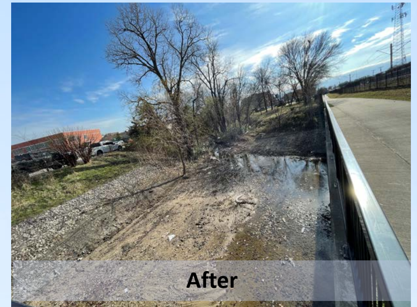
Texas Street Channel
