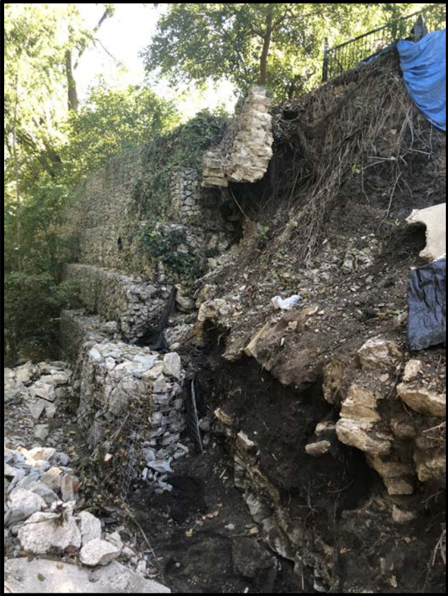
West Fork Gabion Maintenance
