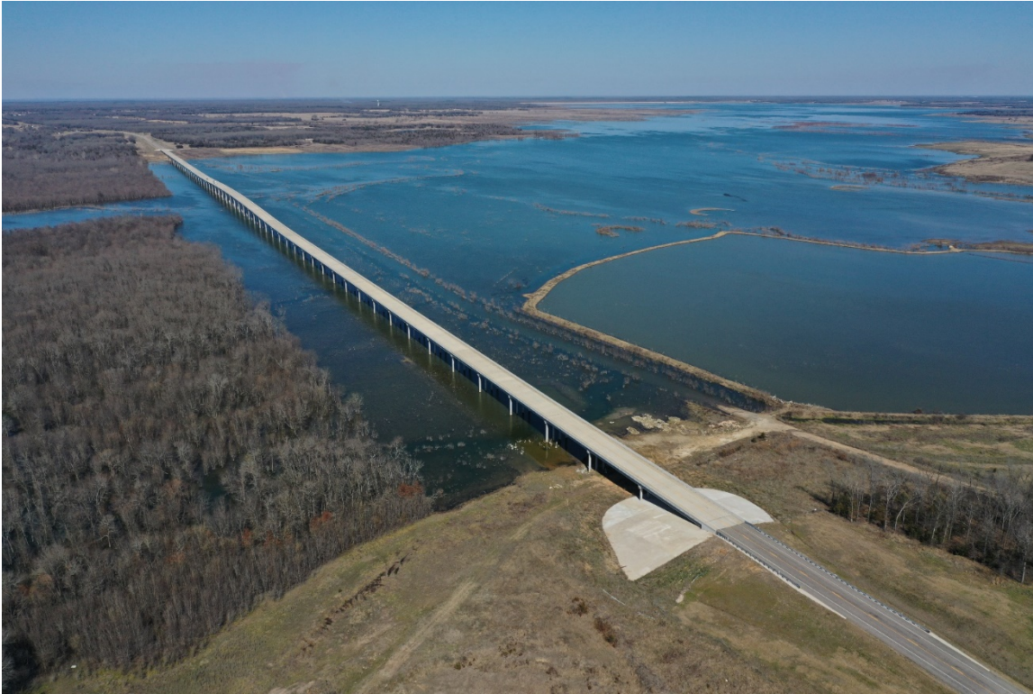
FM 897 Bridge Complete and Open
