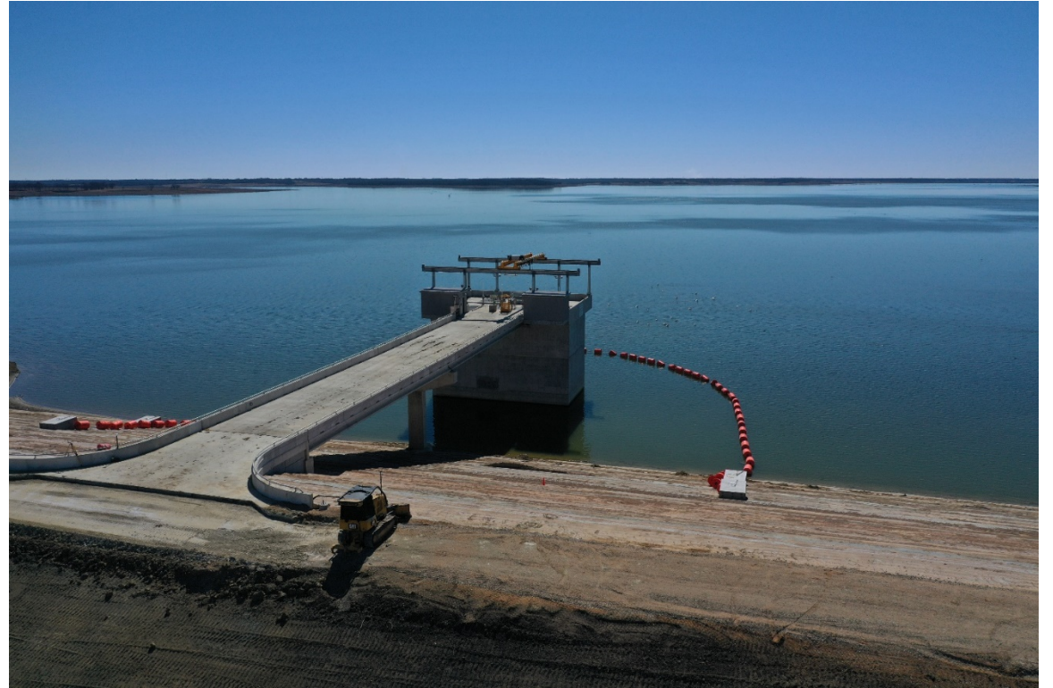
Intake Tower Construction and Wet Side Impoundment
