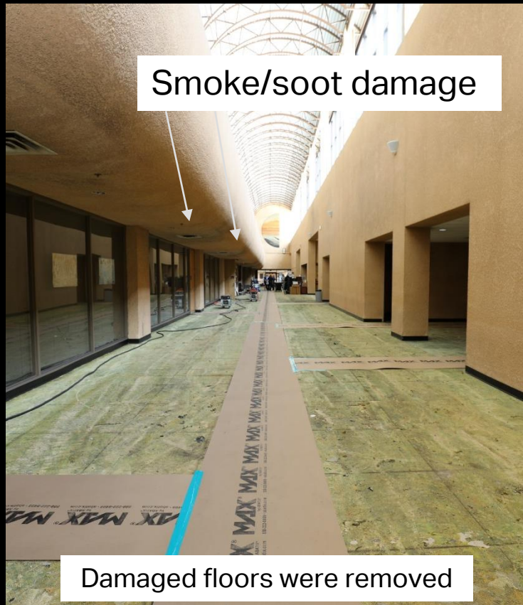
Main Concourse – East End
