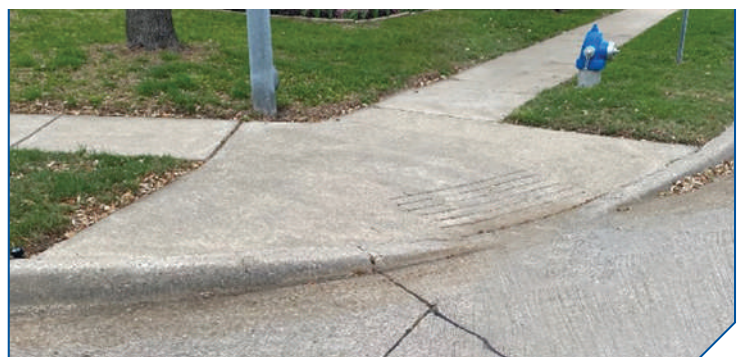
Non compliant Diagonal Ramps
