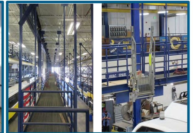
Upgraded Fall Protection for Increased Roof Access Work
