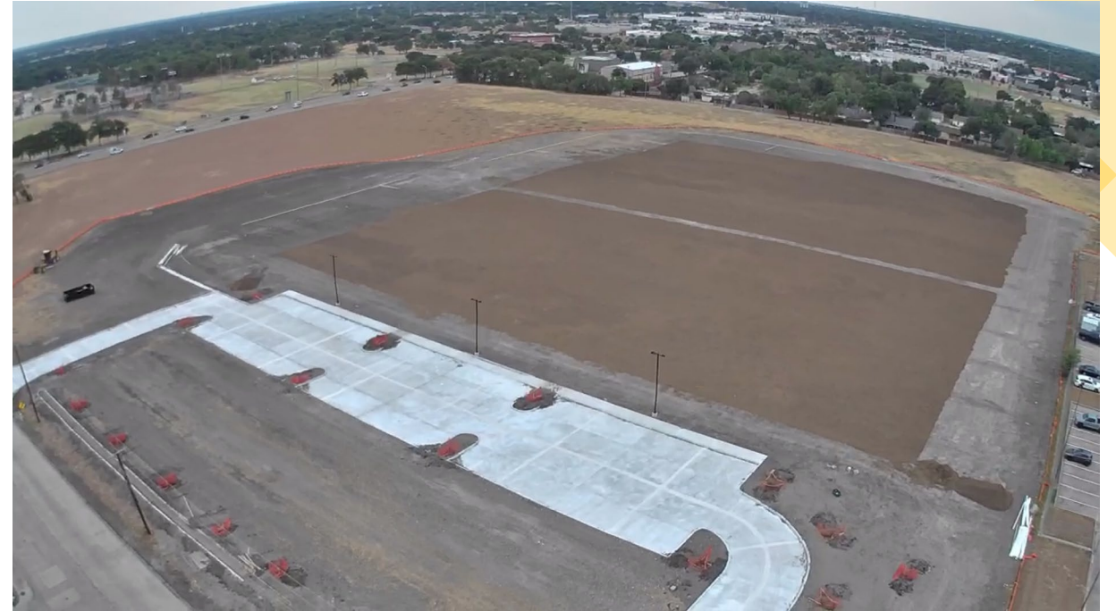
Aerial Site Photo Prior to Grass Seeding
