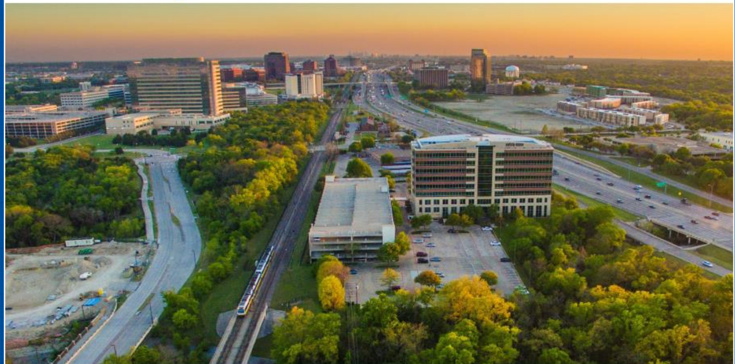
US 75 and Renner Looking South
