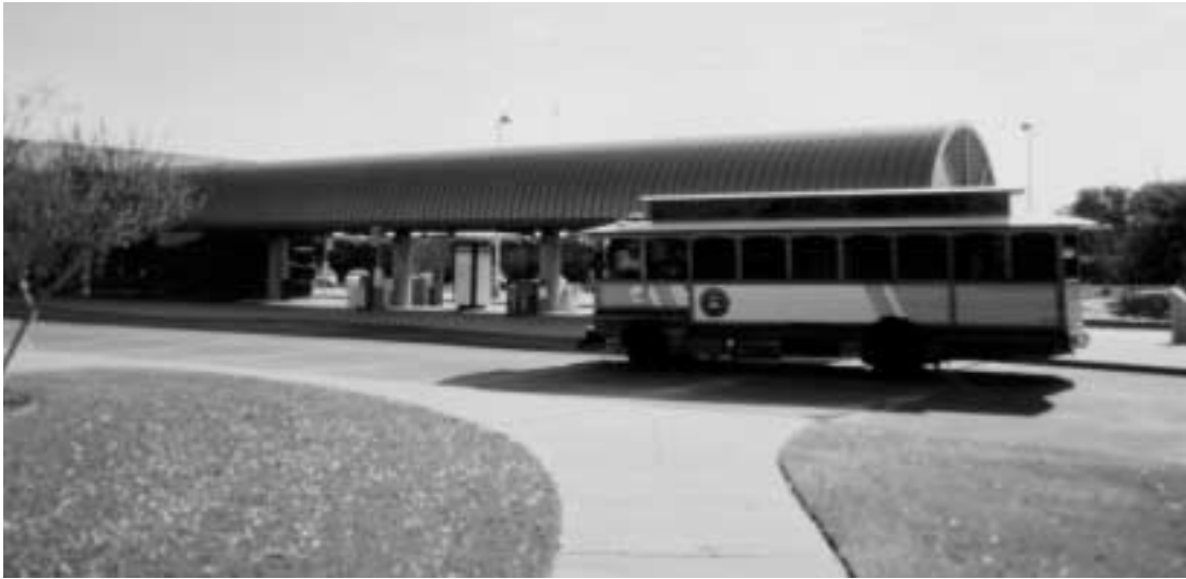
The Arapaho Center light-rail station is located next to the Arapaho Transit Center, which serves 16 routes in the greater Richardson area with buses, including this trolley bus.
