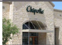
+ SIMPLE Signs should be simple and scaled appropriately to the building's proportions.
