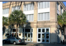
+ PARKING STRUCTURES Doors at the ground floor may access the garage functions or lead directly to commercial spaces.
