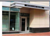
+ SIGN PLACEMENT Signs may be placed in a designated "channel" in the canopy, as well as on storefront glass.
