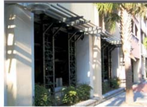
+ MODERN EXPRESSION Metal arbors - not traditional awnings - can help add ornamentation to buildings as banal as parking garages.
