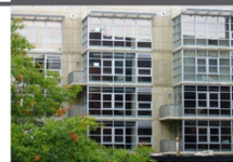
+ WINDOWS OF LARGER BUILDINGS Awning windows in a wall of fixed lites permit modern facades and natural ventilation.
