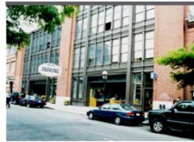
+ CLARITY FOR UTILITY SIGNS Simple, colorful signage can assist with circulation management and wayfinding.
