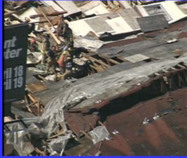
Houston Building Collapse 2009
