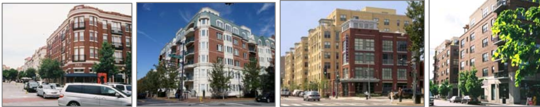
Images showing appropriate building materials within TOD Core, TOD Mixed Use, Arterial and Highway Mixed Use.
