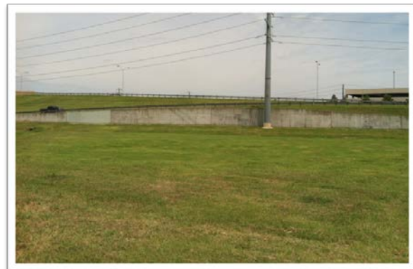
Looking north from site to the grade separated Collins Blvd.
