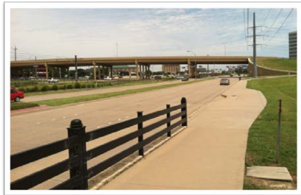
Looking north along Greenville Avenue from the site
