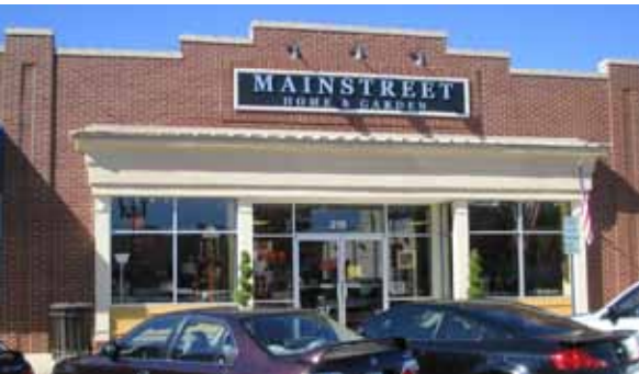
Retail Building on Main Street
