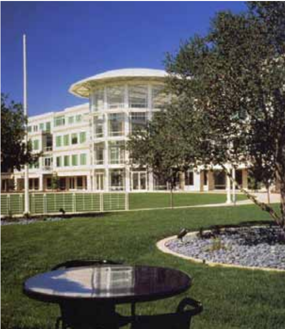
Corporate Office Building
