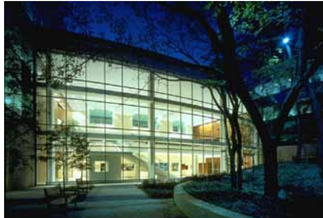
Corporate Office Building
