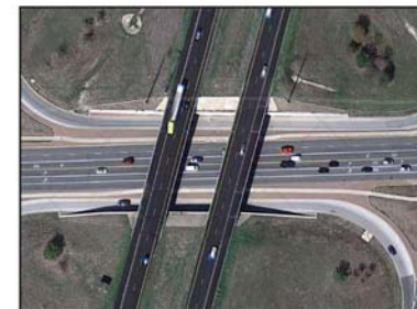
Protected pedestrian access under Central Expressway
