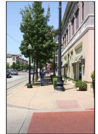
Lighting and ADA Ramps
