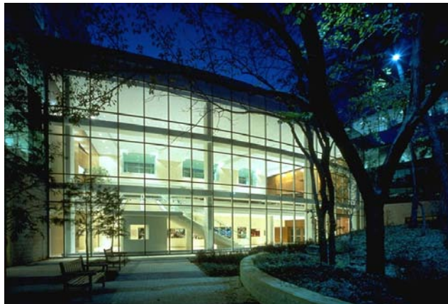
Corporate Office Building
