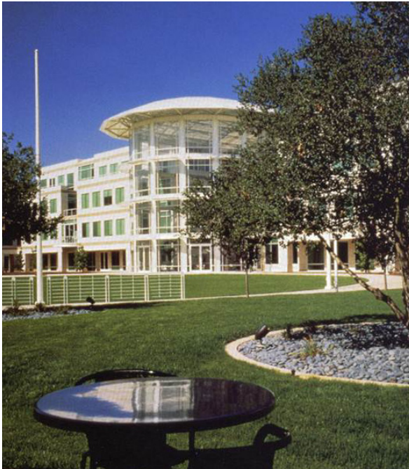
Corporate Office Building
