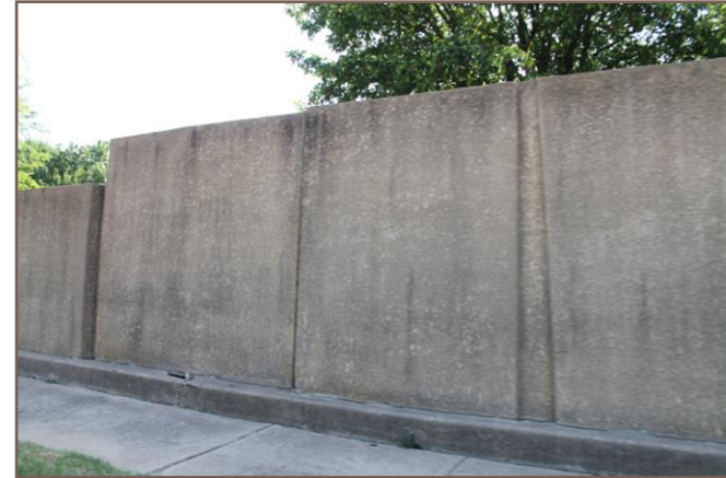
Jupiter Rd (east side) Equestrian Center north to North St. Andrews
