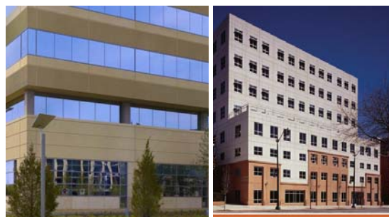
Images showing appropriate use of architectural precast concrete panels as primary building materials
