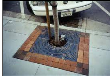
Example of a tree well with a tree grate
