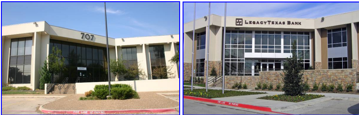
707 E. Arapaho, before and after
