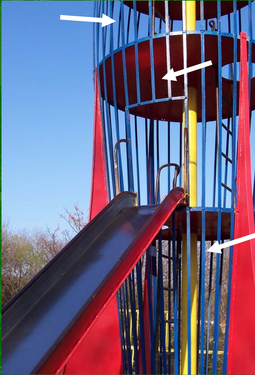
Head Entrapment... between each pair of rails
