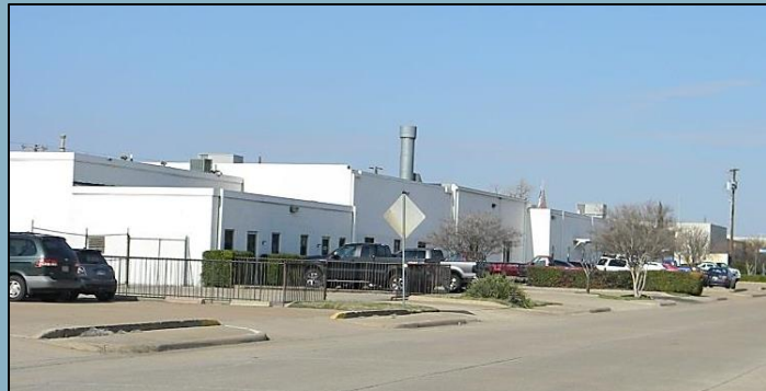
Existing buildings – west side of Interurban St., south of Davis St.
