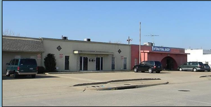
Existing buildings – west side of Interurban St. north of Jackson St.
